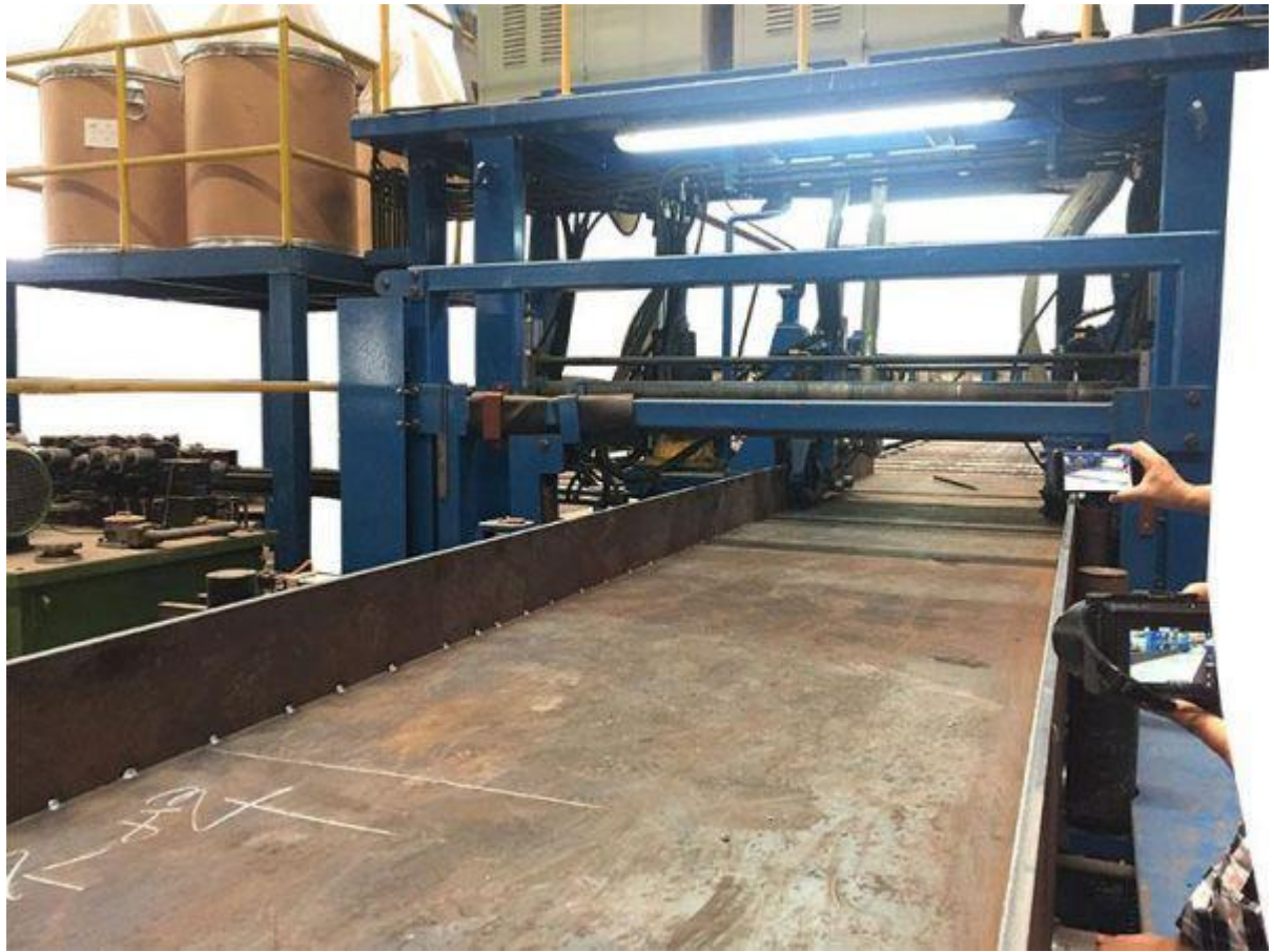
Welding H beam in horizontal position
